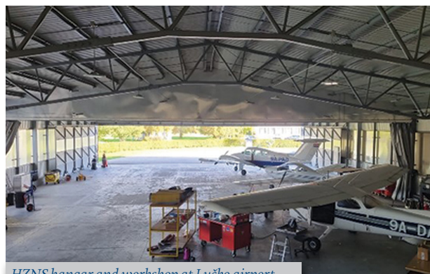
HZNS hangar and workshop at Lučko airport
